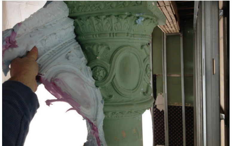
On-site mold removal
